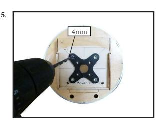
Then, use 5.5mm drill bit to enlarge the holes on the electric motor box.
