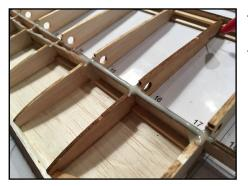
The excess resin, can now be used to glue the top spar into the rib recesses.
