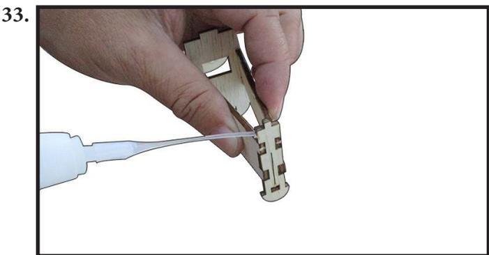
Locate and assemble F5B to fuselage by CA glue as photo shown (photo 37).
