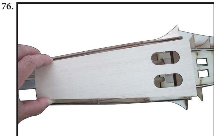
Locate and apply double 8mm balsa F8A to fuselage (left side and right side) by CA glue as photo shown (photo 77).
