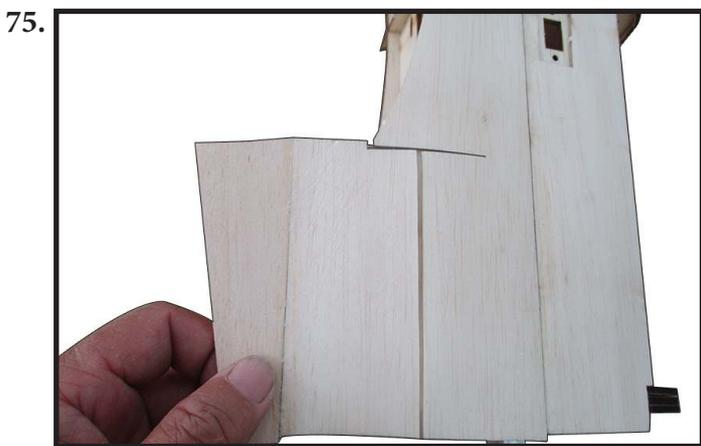
Locate and apply the sheet SH11 to fuselage by CA glue as photo shown (photo 76).
